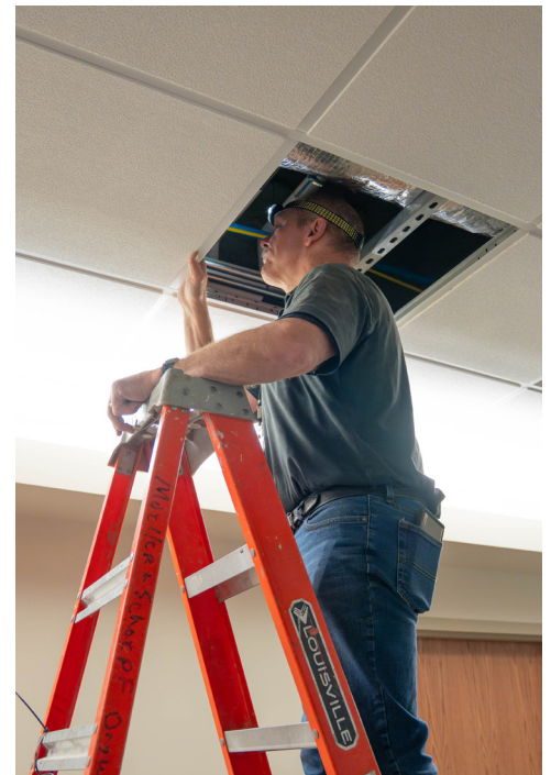
Maintenance engineer Robert Sandifer inspects above the hospital's ceilings.
